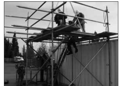
(Left) Tyler Parcha, entrant, dons the supplied contained breathing air tank over his personal fall arrest system preparing for the possibility of a “rescue.” (Middle) Entrant ascends to platform point of entry and supplied air attendee, Jane Brown, readies for the retrieval. (Right) Entrant prepares to shove off stationary platform and be suspended entirely dependent upon the rescue system.
