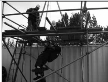
(Left) Rescuing entrant is lowered in suspension into the IDLH situation for rescue. (Middle) Getting a person stabilized and controlling their free motions during their suspension, (Right) they still need to get him through the hole, get him released, stabilized, disconnected, and out of the way.
