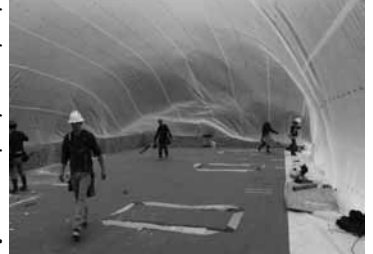
Carpenters working on the Juneau City Shop-North Pacific Erectors
